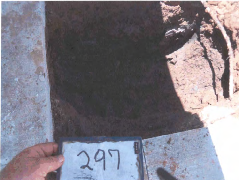
Picture 2: UST 297Birch excavation.
